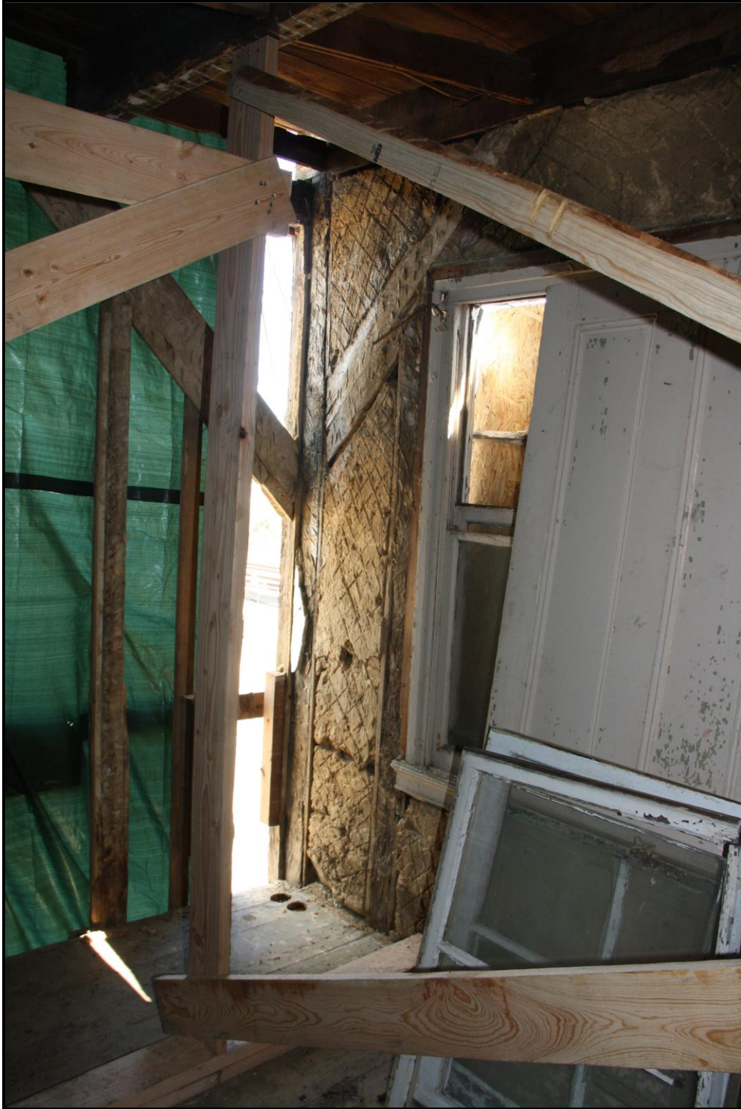
View Northeast inside the T. Thomas Fortune house showing clay wall nogging.
