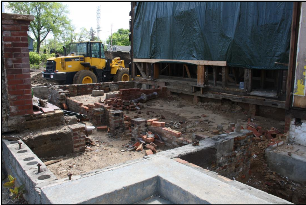
Rear of the Fortune house following the removal of 20 th century additions. The brick foundation within the concrete block foundation may indicate the location of one or more earlier additions.
