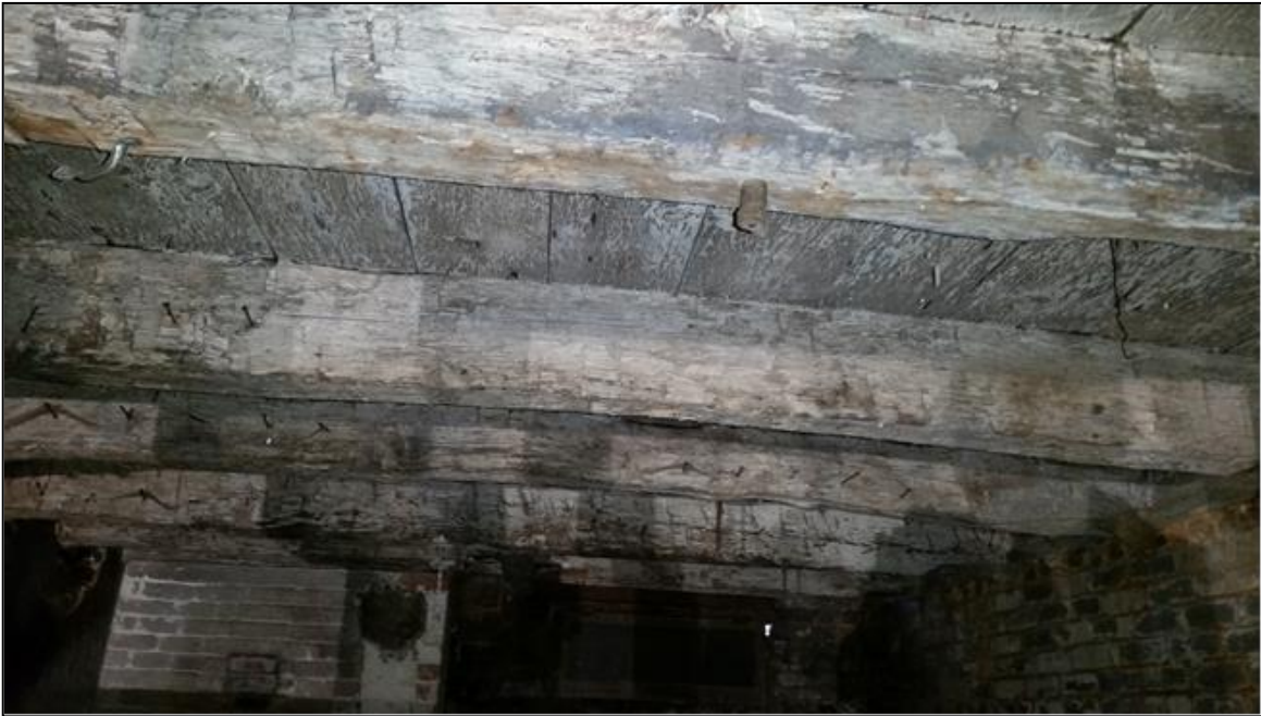
View looking east in the cellar of the main block of the house showing the joists supporting the first floor and a brick fireplace/chimney support.
