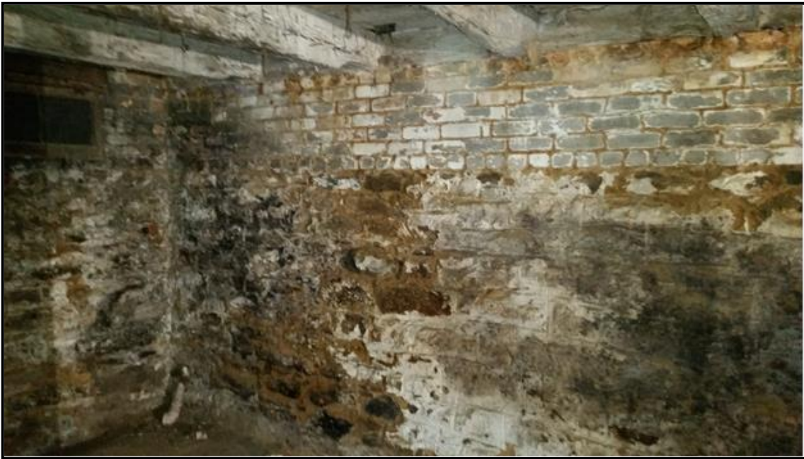
View looking southeast in the basement of the main block of the house showing the original rough stone foundation, overlain by the brick foundation and the timber joists supporting the first floor.
