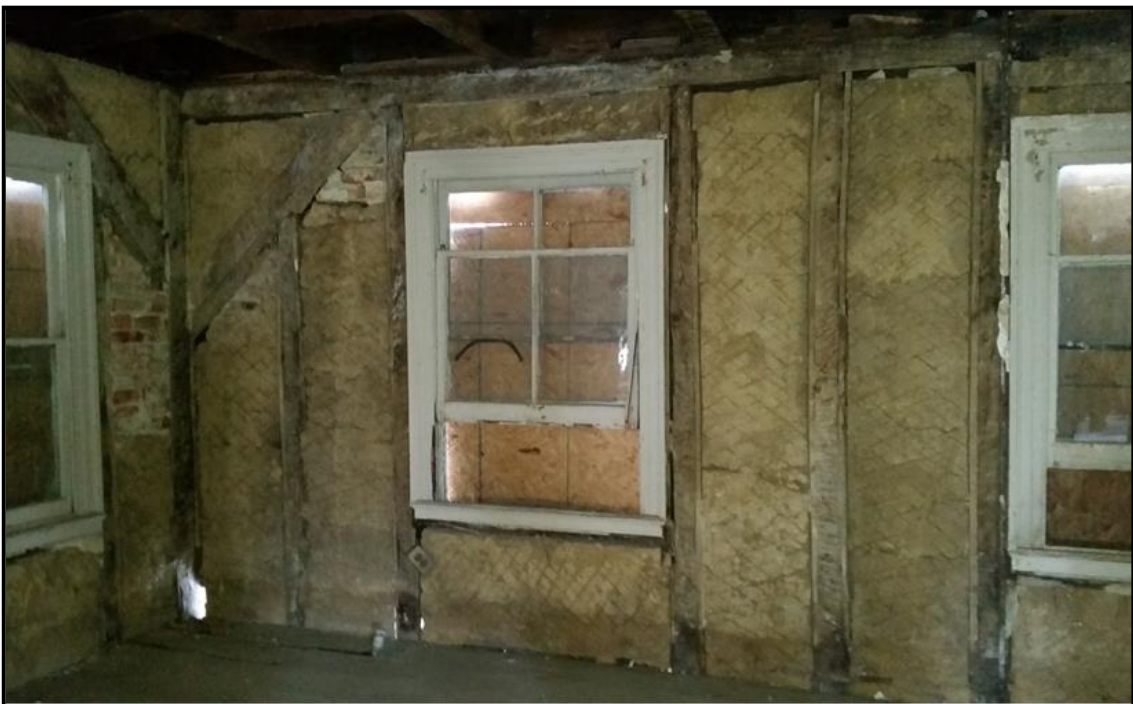
View south, showing the south wall and southeast corner of the main block of the house on the second floor. Note the timber framing, with clay noggin in the walls. The clay is scored to take a rough coat of plaster—now removed.
